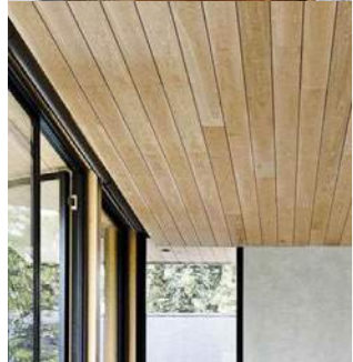
4 Timber ceiling to entrance
