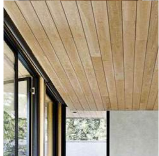
4 Timber ceiling to entrance
