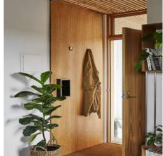
3 Timber entrance door
